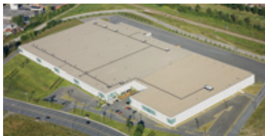
Reitmans Distribution Centre, Montreal, Québec
