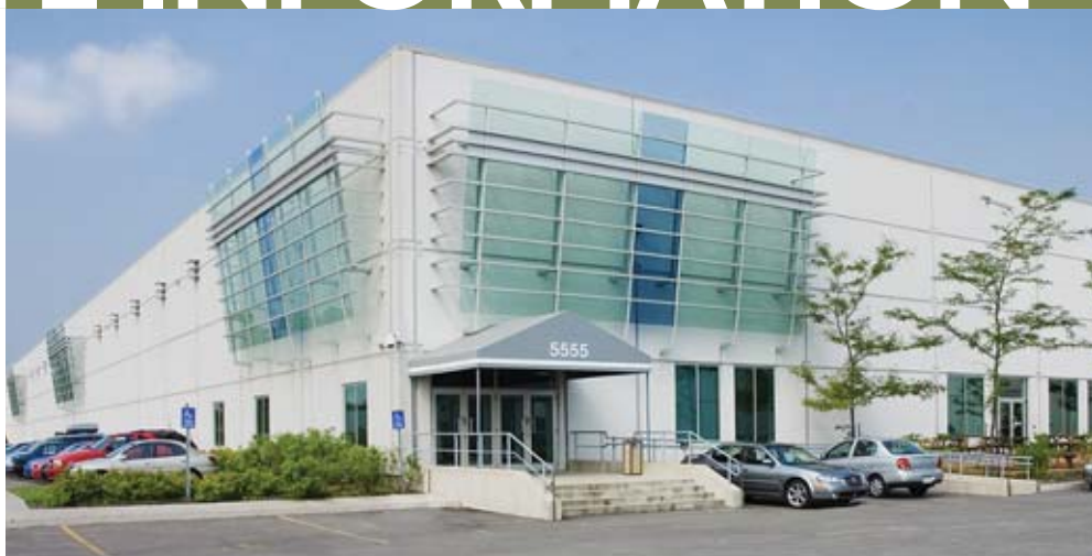
Reitmans Distribution Centre, Montreal, Québec
